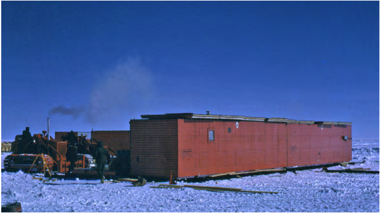
Top: US Navy “Sea Bees” push the main camp sections together January 1966
