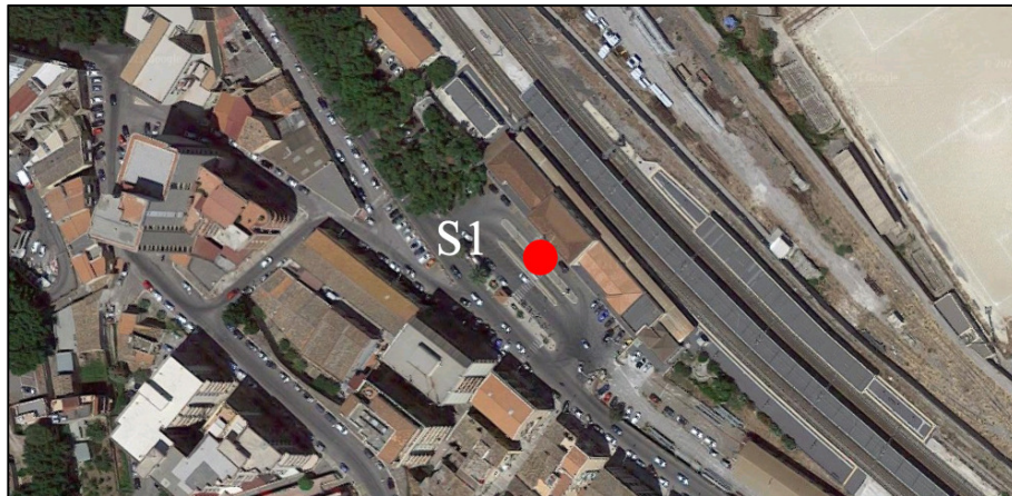
Fig. 4. Borehole location in the municipality of Termini Imerese (PA)
