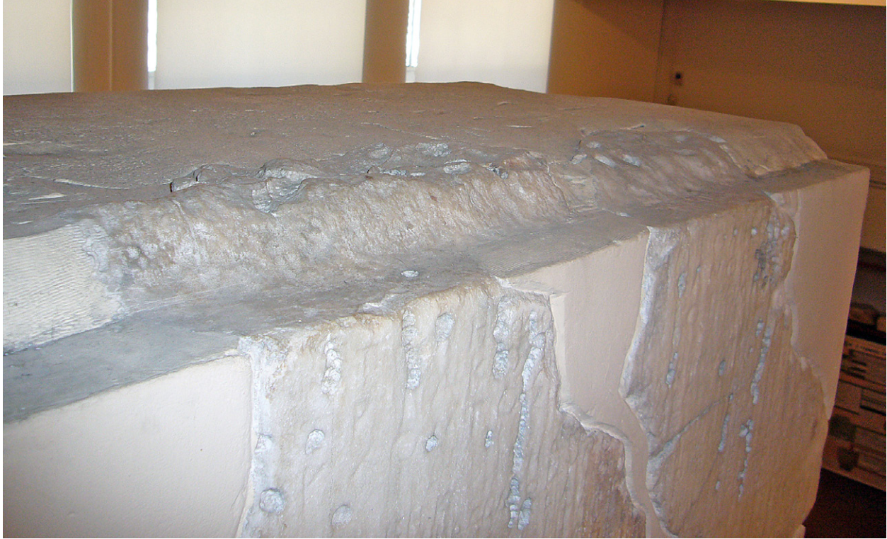
Figure 5. Lapis primus (IGF 259–272), detail of top, showing drafted margin along front side and quarry surface remaining behind
