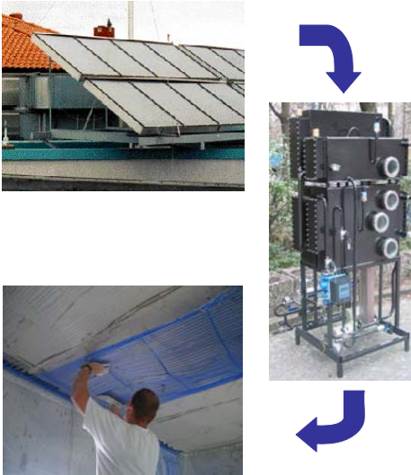
Figure 6 – Low temperature lift system: Low exergy cooling system using chilled ceilings, a low temperature driven single effect absorption chiller (LiBr-water chiller from company Phönix Sonnenwärme) and a flat plate collector
