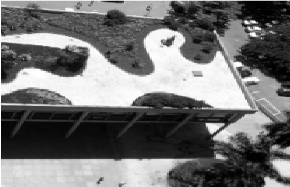
Image 1: Intensively Greened Roof in the City of Rio (MEC), designed by Burle Marx in the 1940s
