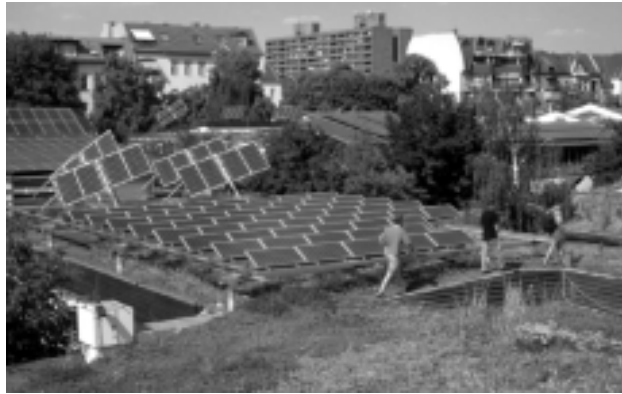
Image 2: (left) Extensively Greened Roof in Combination with Photovoltaic Panels, UFA, Berlin
