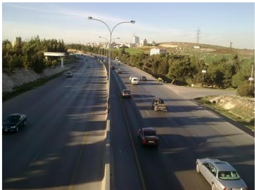
Figure 6.15 Airport Road/Informal public space
