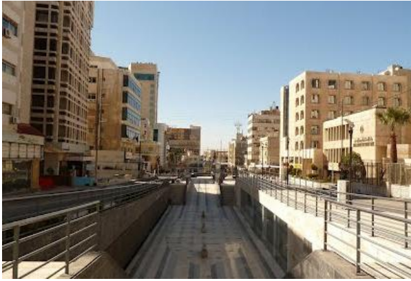
Cultural Avenue, Al Shmeisani
