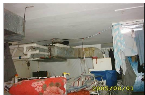
Figure 12 Using Service rooms as accommodation
