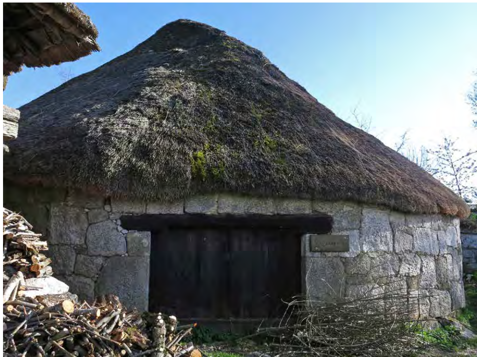
Figure 4: Round structure with hayloft thatched with rye straw (type III) at Piornedo, Lugo. (© Lucía Ruano).
