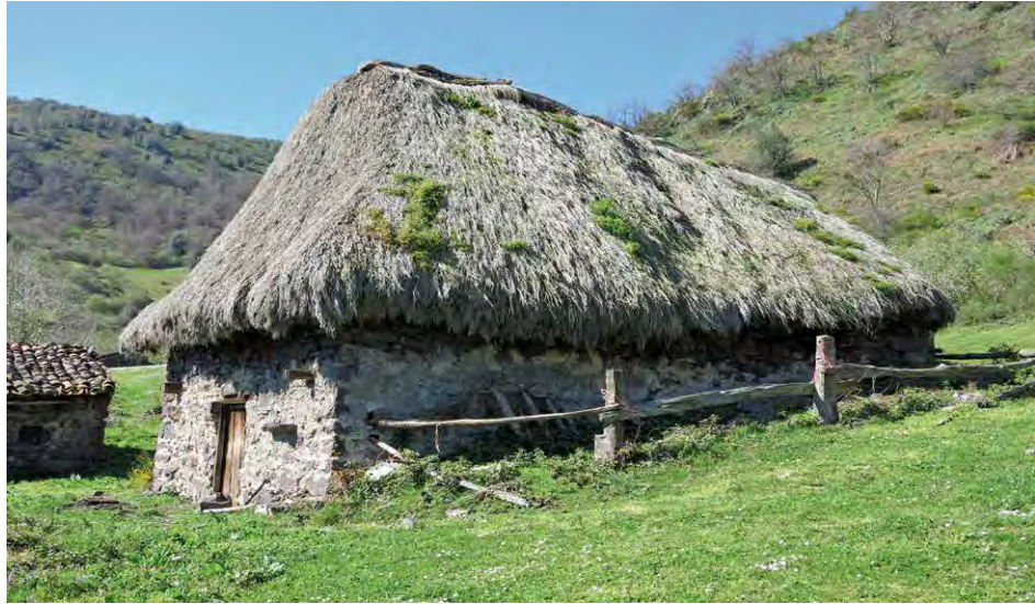
Figure 3: Structure with hayloft thatched with broom (type II) at Teverga, Asturias. (© Lucía Ruano).
