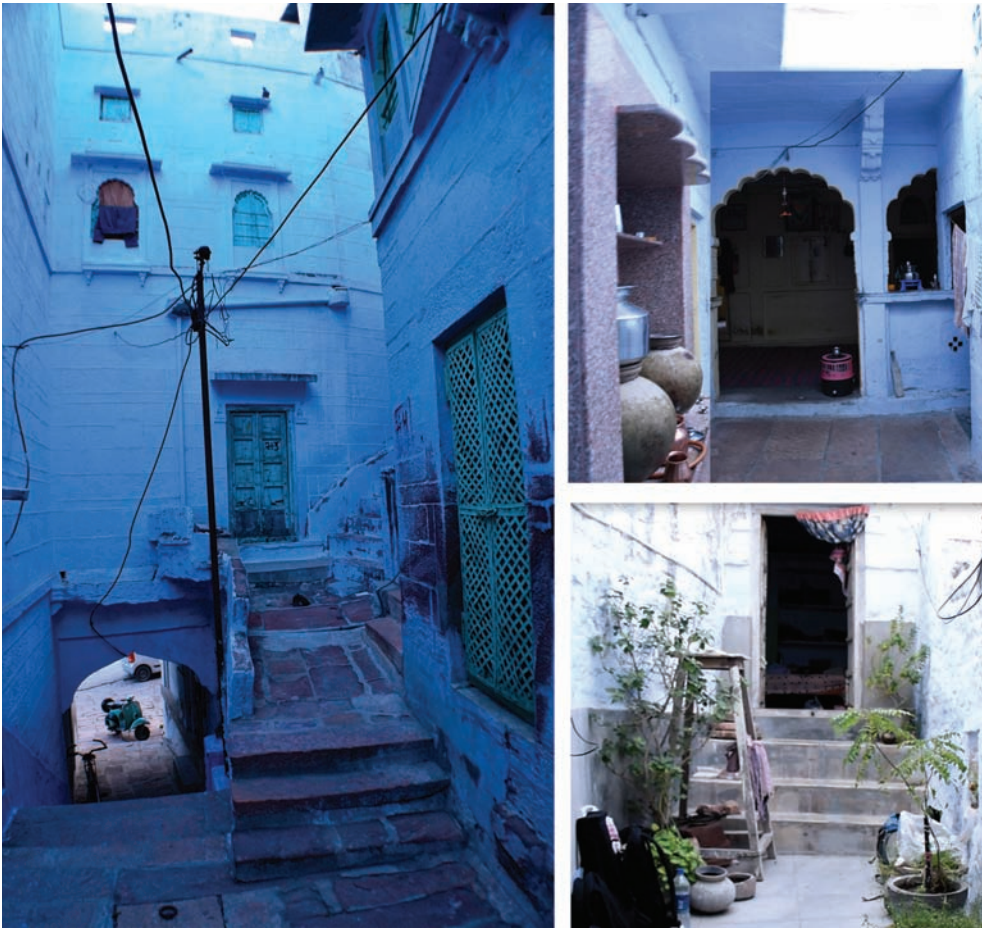
Figure 9: (left) view of the internal street from the Gate and (right) views of the internal courtyards of haveli 1 and haveli 2. This serves as a complete private area
