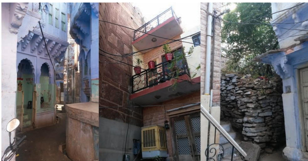
Figure 7: the three images shows typical cases of over-volumes present in the areas. It is possible to distinguish (middle photo) the Fort walls and how the new building growth on it. As previously said the situation of growth of the size of the building is moving towards the vertical direction due to the lack of space along the streets. However, the growth has a very high factor with an average of 64%. This creates high-density areas)
