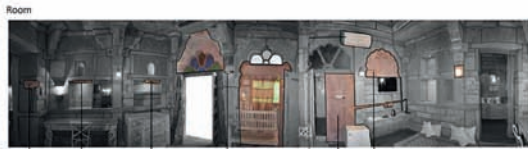
Room Adjustment Done For Hiding Wiring Led Lighting A.C. Unit Additional Wall for Wiring And To close The Bathroom
