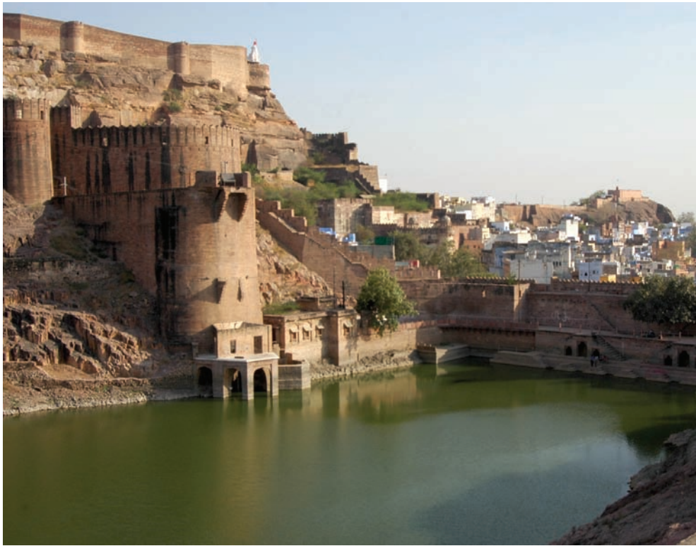
Figure 2: Ranisar This reservoir, created by an embankment below the Fort provided water to the palaces
