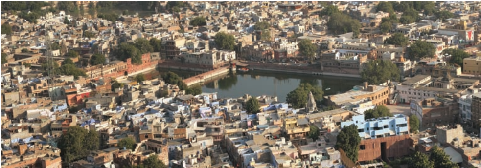
Figure 4: (top) An aerial view of the Jodhpur Historic City with Gulab sagar and Baccha Jhalra. Photo credit Sanket Mhatre
