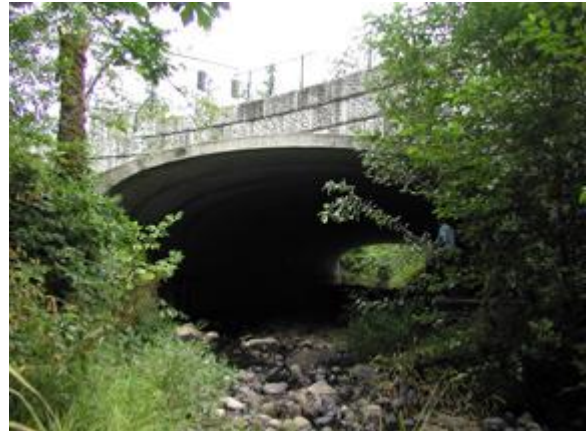
Figure 7. The Lakeside pedestrian and wildlife undercrossing in Portland, Oregon.
