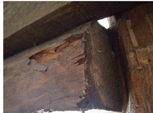
Figure 4: Details of the infestation by *C. brevis* in Rua da Junqueira, Lisbon. Termite fecal pellets on the floor and aspect of an infested timber beam.
