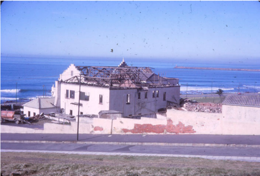
Figure 6. The Beach Hotel in the process of demolition.
