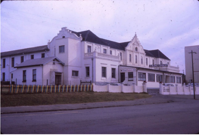
Figure 5. An image of the Beach Hotel while still in operation.
