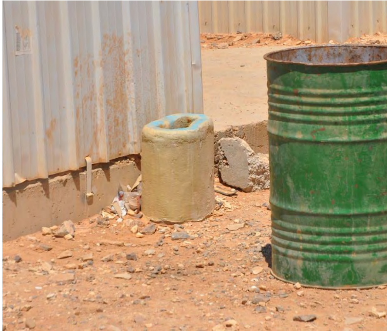
Image 10: Commode-style toilet, removed from accessible (ramped) cubicle, Al Azraq Camp, Jordan
