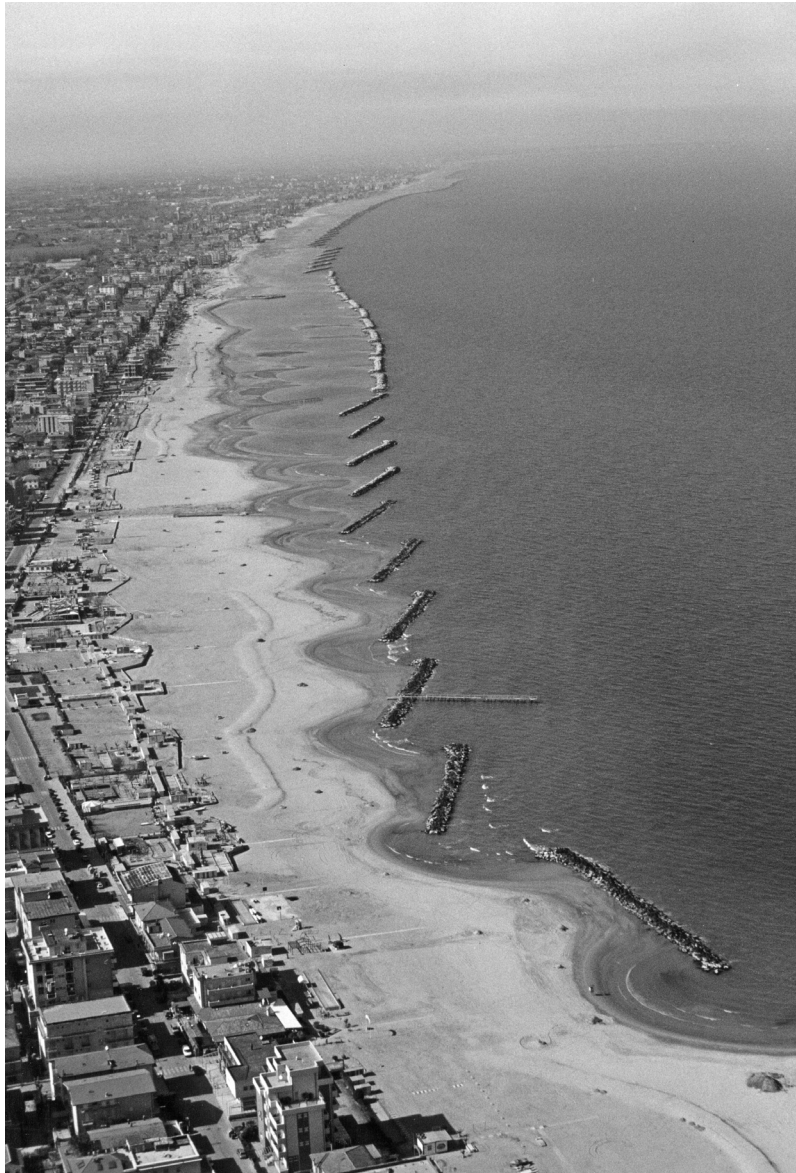
Figure 5 Coastal defence structures along the highly urbanised Italian shores of the north Adriatic Sea. (Photo by Giorgio Benelli. With permission.)
