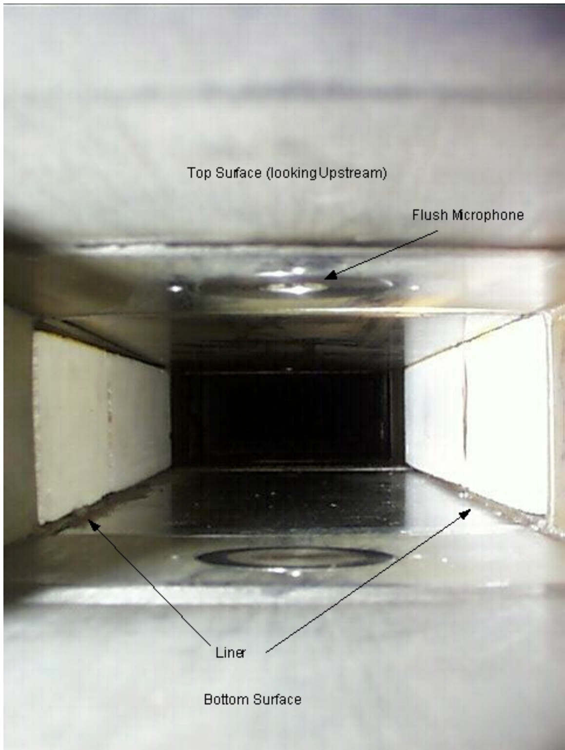
Figure 15b. Photos of flow duct with liner installed on side walls (looking upstream from exit).
