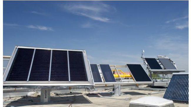
Figure 1: Testing facilities of the TestLab Solar Thermal Systems, Fraunhofer ISE
