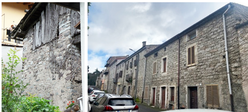
Figure 2: Facades of small historical centres built with local materials. On the left, Storo (I), with its typical constructions in stone and timber. On the right, Buddusò (I), with houses built in grey granite blocks.
