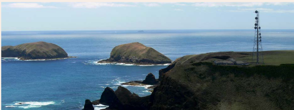
Cape Grim Baseline Air Pollution Station, Tasmania, situated 90 metres above sea level Photo by CSIRO, CC BY 3.0
