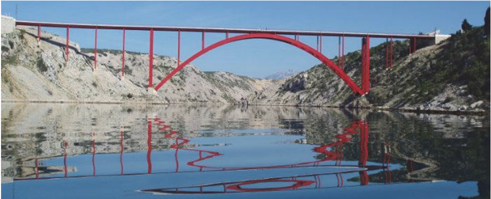
Figure 13: Maslenica Bridge on the Adriatic Road
