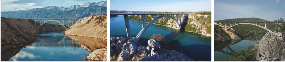
Figure 20: Maslenica Bridge (left), Skradin Bridge (middle) and Cetina Bridge (right)
