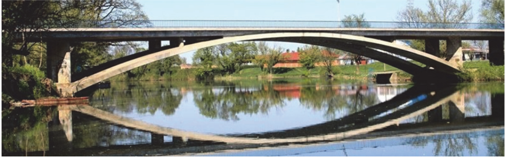
Figure 17: Bridge over Korana River in Karlovac
