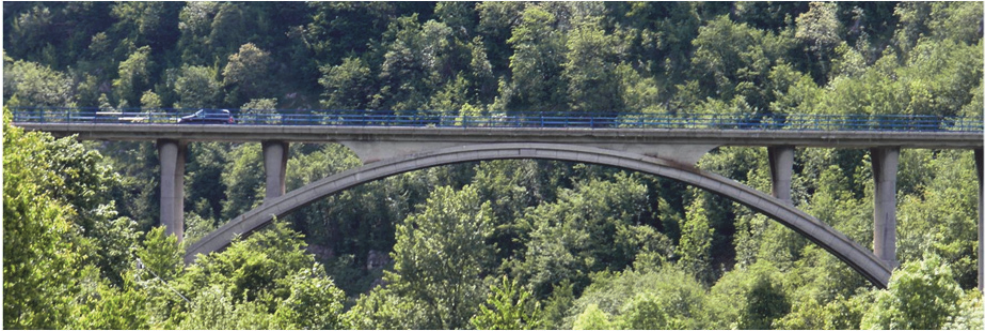
Figure 15: The bridge over Korana River in Selište
