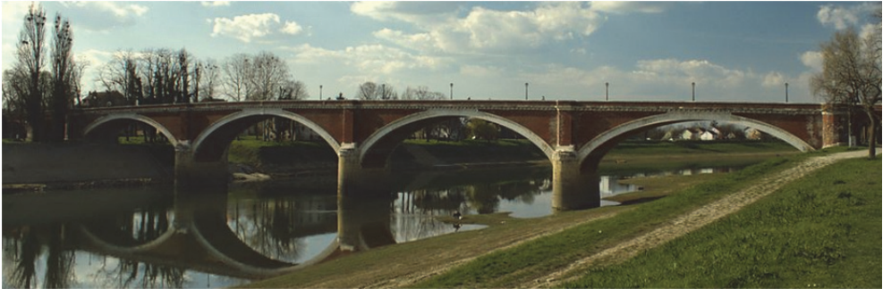
Figure 9: The Bridge across Kupa River in Sisak
