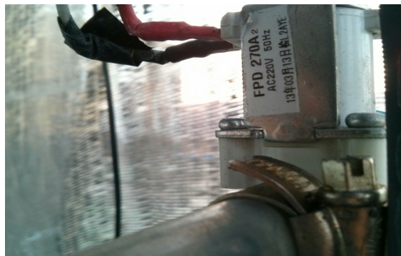
Fig. 7. Solenoid controlled by ultrasonic sensors.
