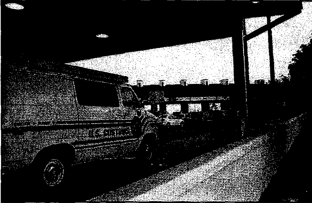
INS toll stations at International Bridge No. 1, Laredo, Texas, March 2000. Scott Cook
