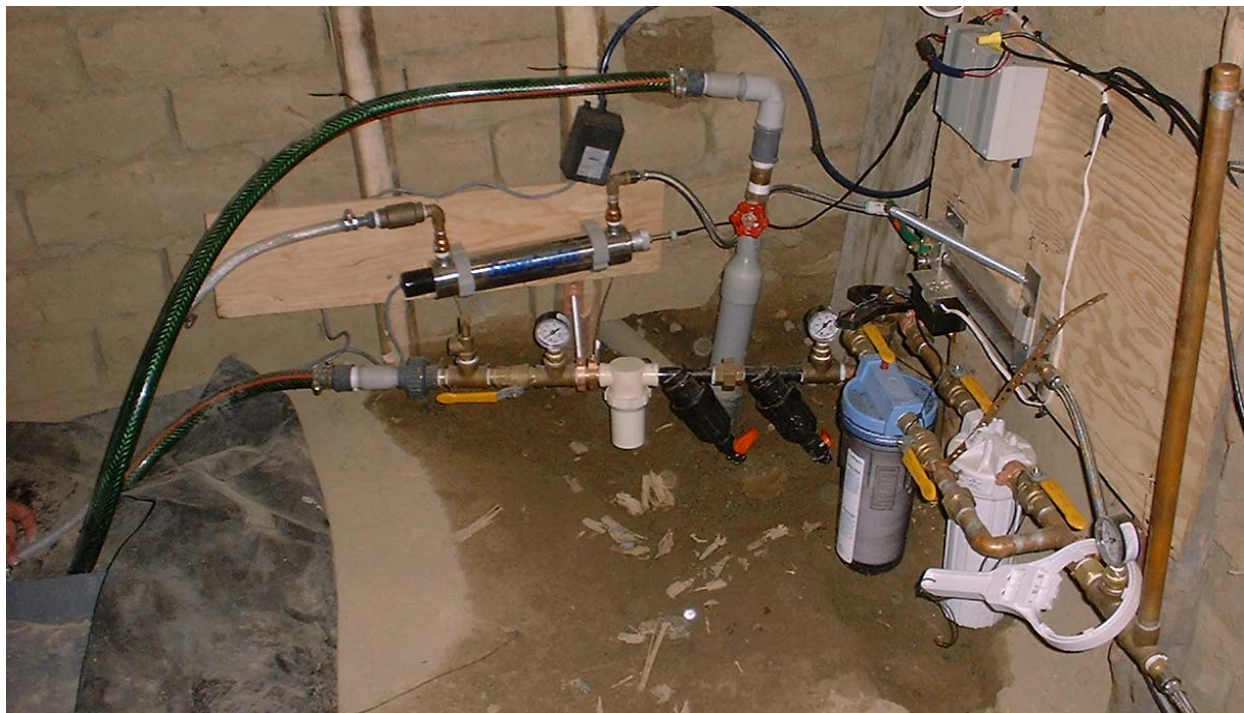
Fig. 4 Part of installed system inside adobe shelter: flexible tank to left on floor, UV light in stainless tube to right of tank horizontal on plywood (near center of photo), filters below and to the right, failsafe shutoff valve mounted to bottom of plywood on the right just above filters.
