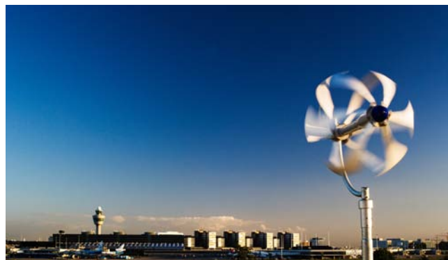
Fig. 1. Venturi wind turbine installed at Schiphol airport Amsterdam, The Netherlands.
