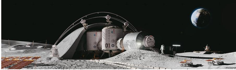
**Figure 1:** Rendering of six MaMBA modules and an airlock on the Moon covered artificial cave.
