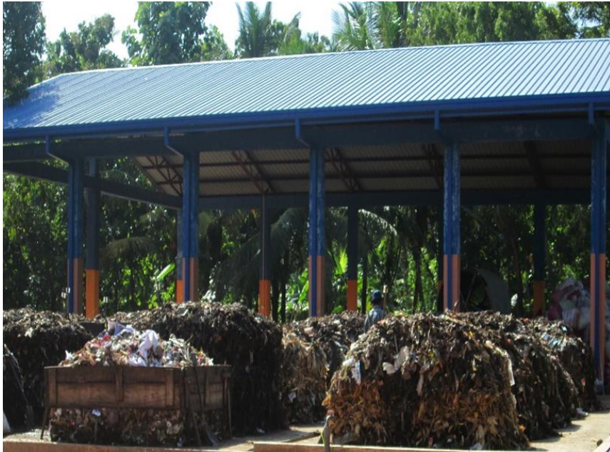
Wariyapola Compost Plant (Source: IWMI)
