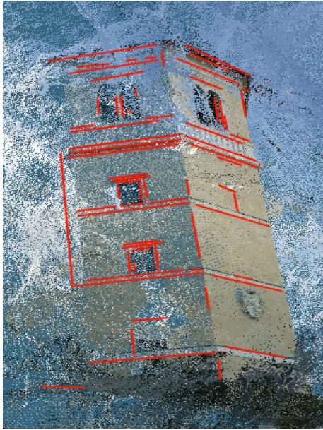
Figure 1: Fusion of automatically extracted 3D lines and 3D point cloud. The illustration shows the bell tower on the castle hill in Graz.
