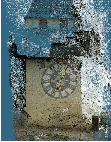
Figure 5: 3D point cloud of the clock tower on the castle hill in Graz.
