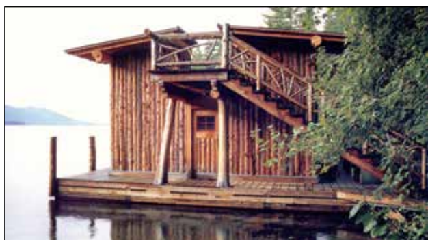
Figure 1. The façade with a final coating of half logs, Winter boat house, Lake George, New York, Architects: Peter Bohlin, Royce Earnest, Robert McLaughlin 1992 [2]
