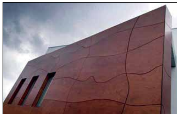
Figure 7. The façade coated with “Prodema” composite plates, Clinica Pombaldial, Lisboa, Portugal, Architect - Filipe Sousa[10]
