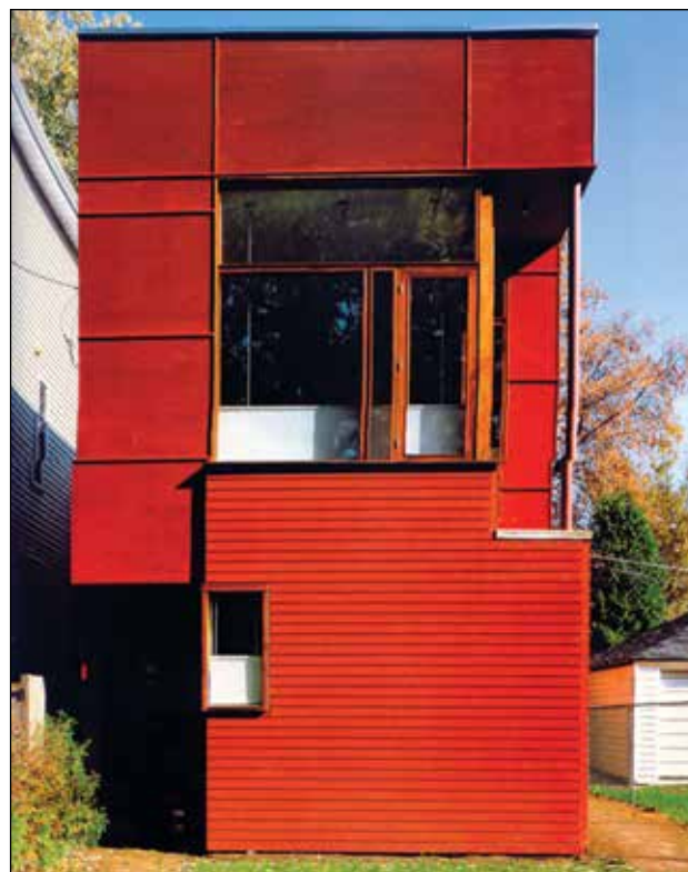
Figure 2. The façade performed in combination of wooden plate cladding and wooden cladding from single elements, House in Toronto, Canada, Shim - Sutcliffe Architects - architectural team, 1994 [3]
