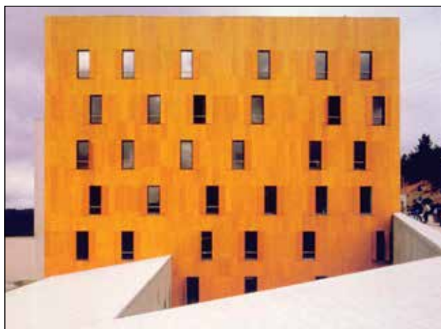
Figure 6. Waterproof veneer panels as façade cladding, Dormitory, Campus II, Coimbra, Portugal, Architects -Manuel Aires Mateus and Francisco Aires Mateus, 1999 [6]
