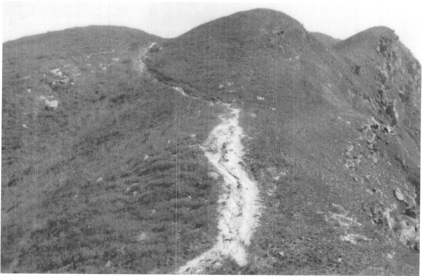
Figure 3. Trails with low slope alignment angles (lower portion of photo) are more susceptible to different forms of trail degradation than those with high slope alignment angles (upper portion of photo)
