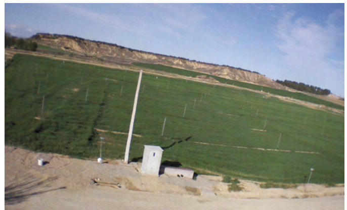
Fig. 2. Aerial video analysis detecting blocked sprinklers.
