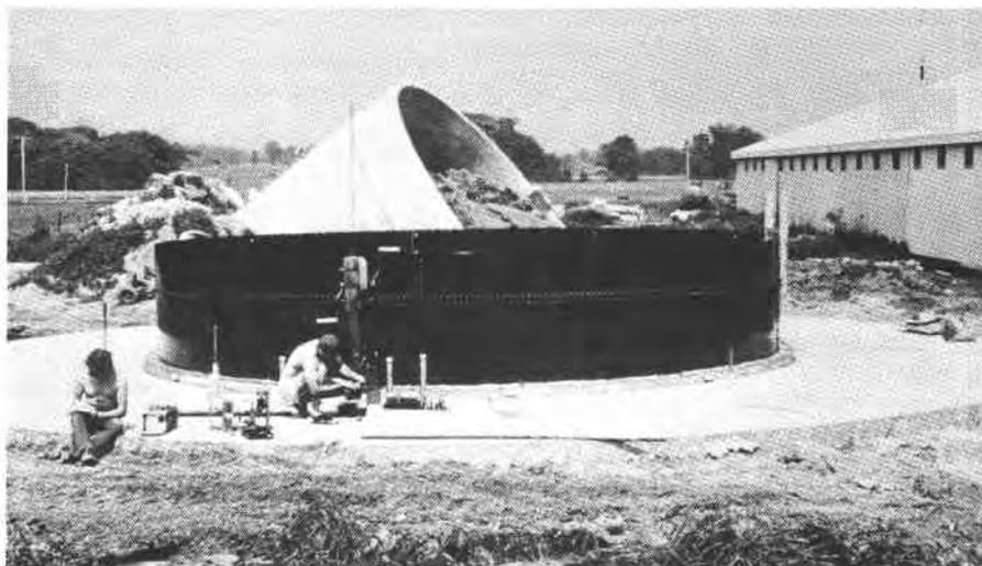
Figure 2. Raft foundation for tower silo. Portion of failed silo in the background.
