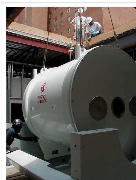
Heavy lifting equipment is used to install the MRI unit.
