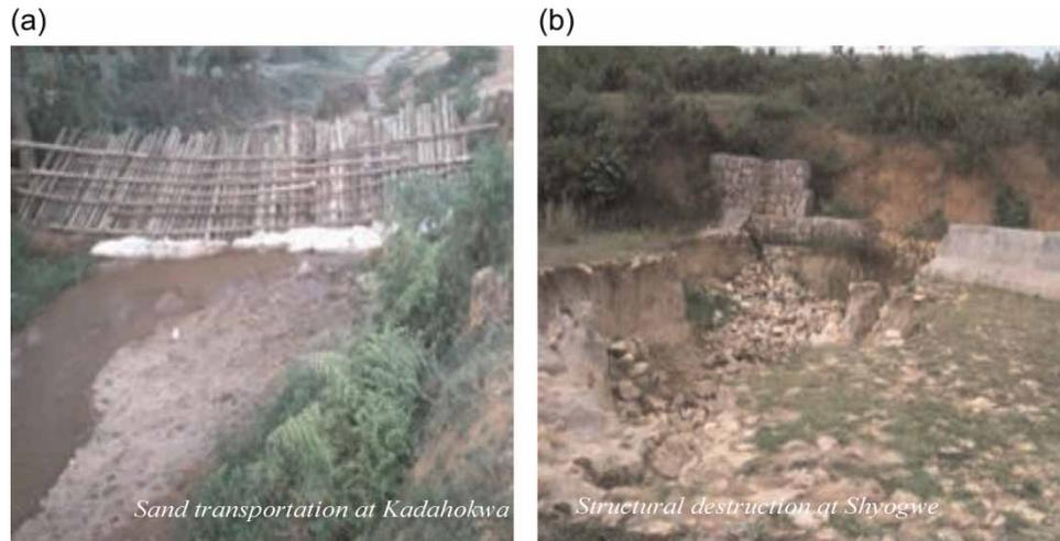
**Figure 10** | Typical problems experienced at intake systems: (a) destruction of sand-retaining structure at Kadahokwa and (b) spillway failure at Shyogwe.
