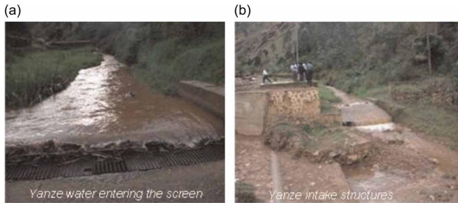
**Figure 3** | Yanze water intake up to the treatment plant.
