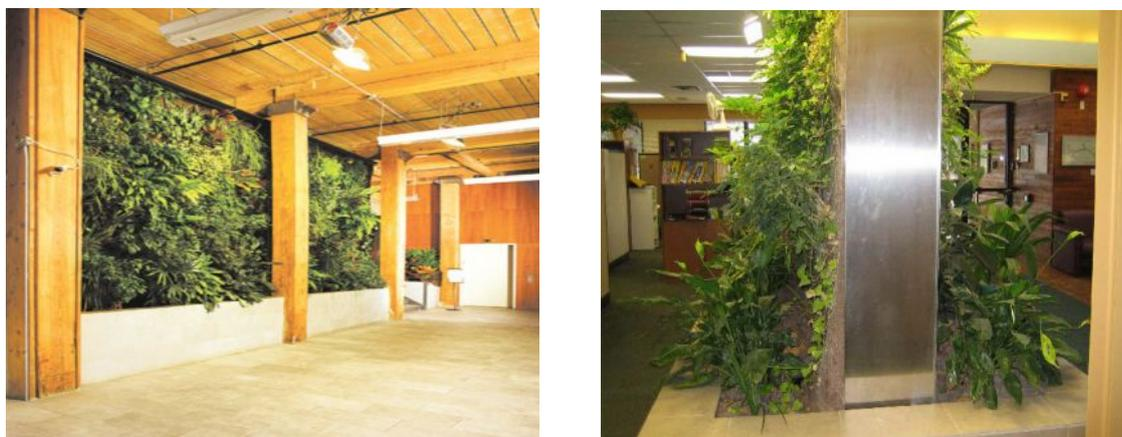
**Figure 1. Biowall for air pollutants filtration<sup>64</sup>.**
