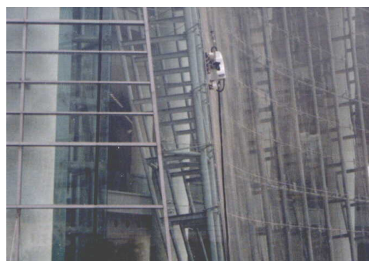
Fig. 7 Sky cleaner cleaning on the target glass wall.
