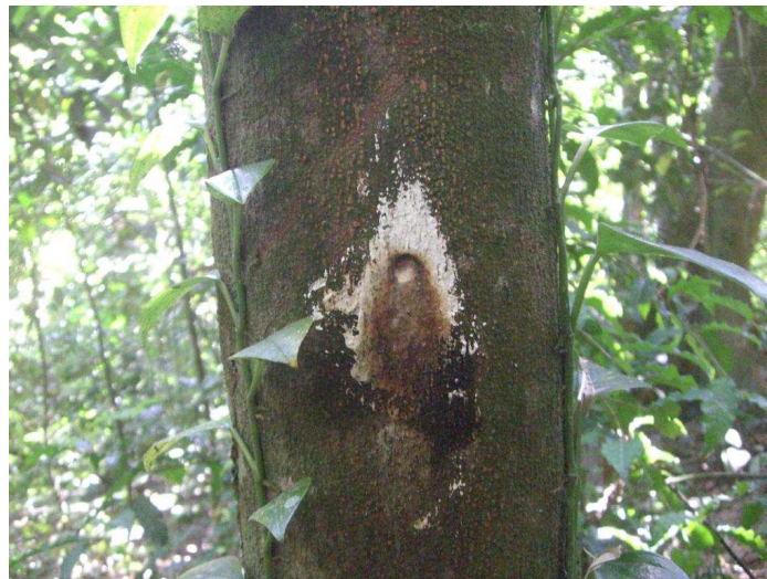
Figure 4 – Hole after the drill. The white color is from the synthetic plaster.
