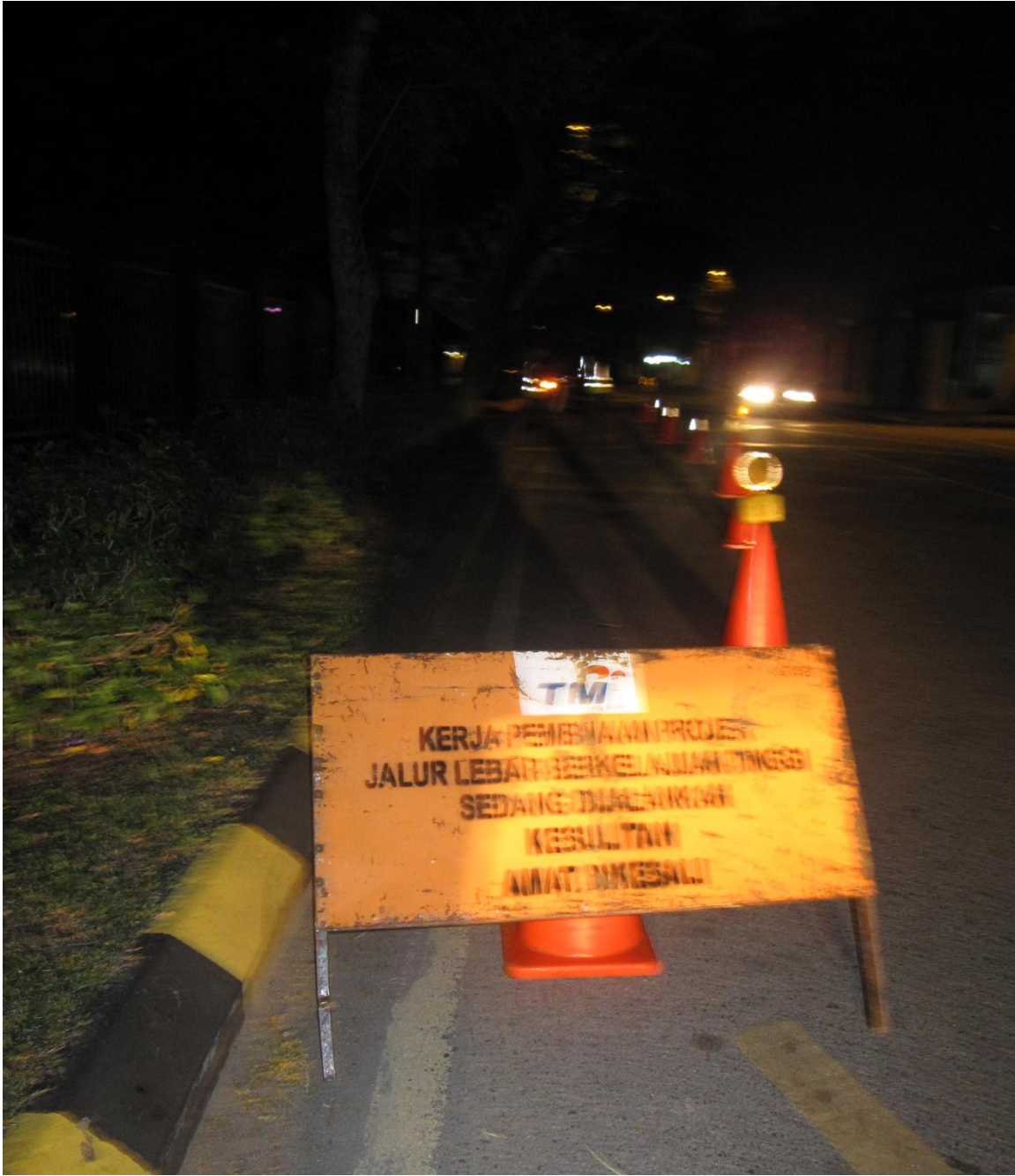
Figure 19: Implementation 2 team night work
