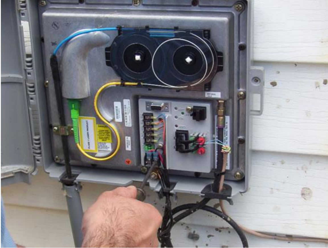
Figure 18: ONU installation 2
