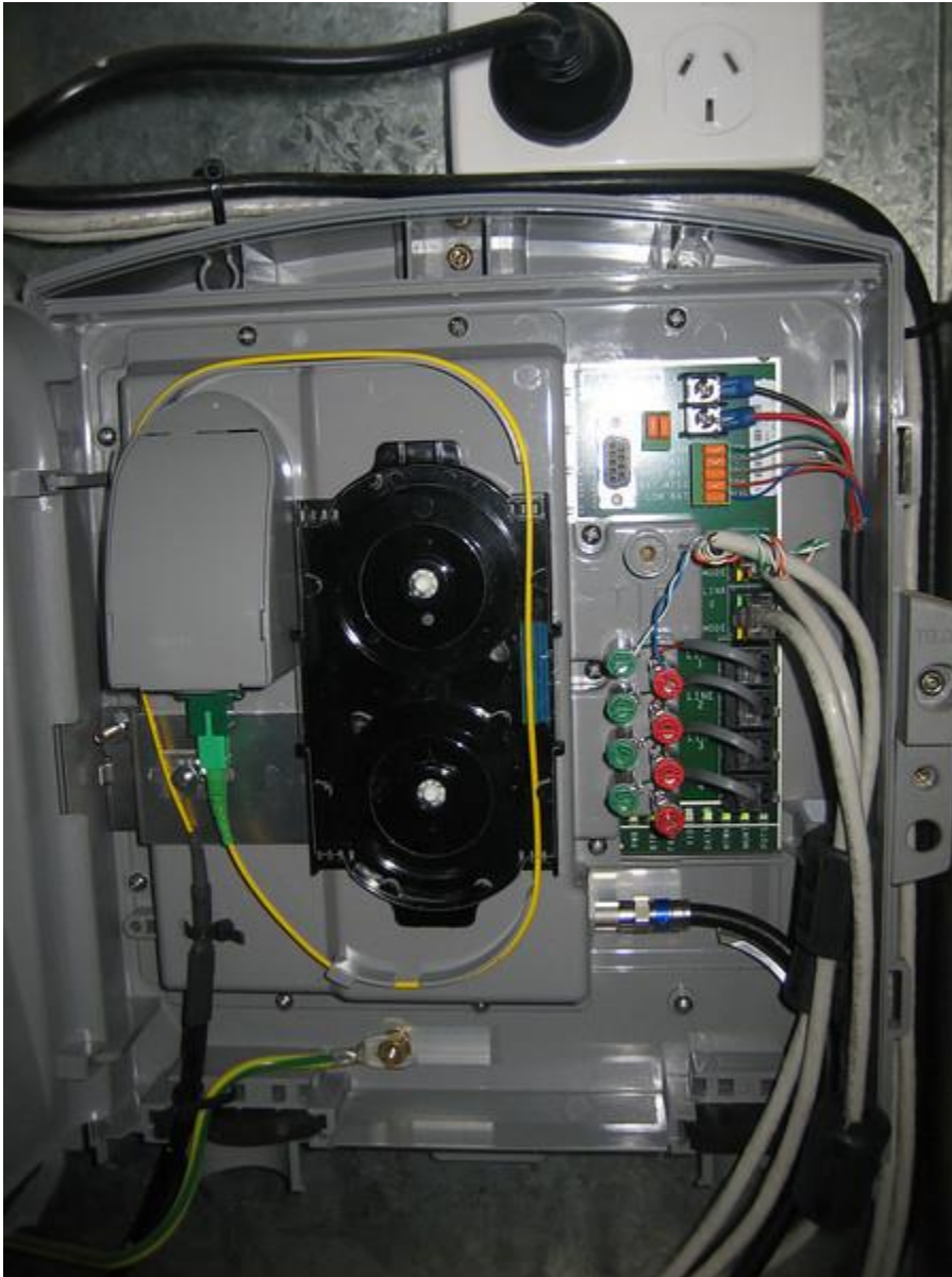
Figure 17:ONU installation
