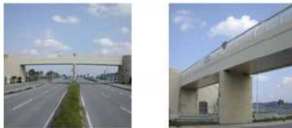
Fig. 42: Pedestrian Bridge in Okinawa, Japan made of Hybrid Composite [51].
