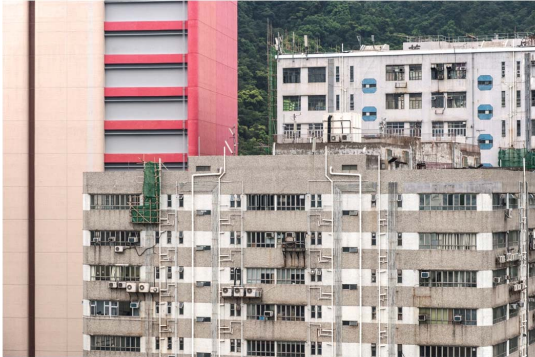
Figure 3. Rooftops. Photo: Stan Diers ( www.standiers.com )
