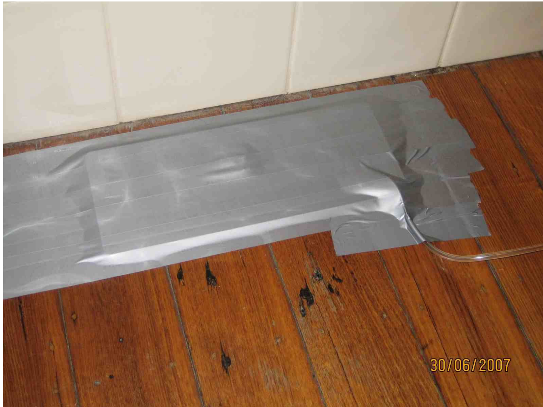
Figure 9 Floor register sealed with duct tape, with tube inserted, which is connected to the pressure gauge to measure pressure within duct system.
