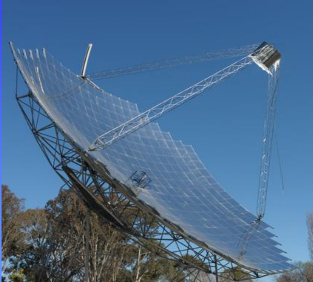
ANU Big Dish parabolic concentrator with steam generation cavity receiver
