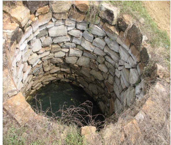
A view of the open well constructed under Mangalpur sub-minor which facilitates conjunctive use of water for irrigation to crops
