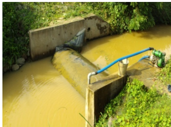
Plate1. Rubber dams installed in watersheds of Odisha by IIWM, Bhubaneswar
