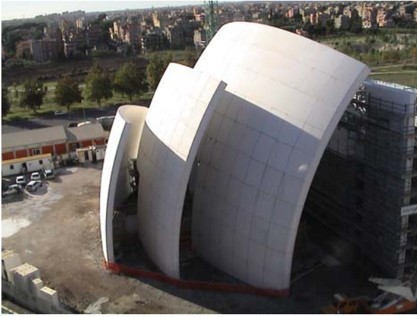
Figure 5. Construction of the Church (sails)
