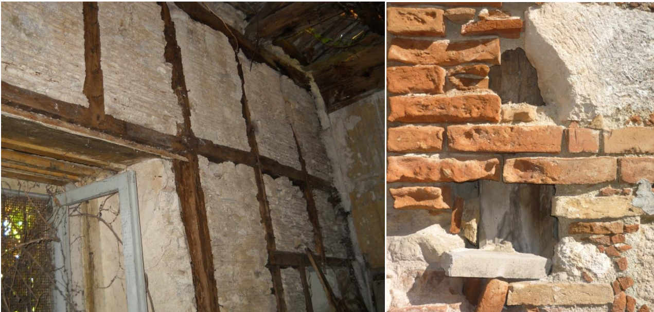
Figure 1. Different types of timber frame arrangement. The framing is placed in the internal (on the left) and in the external part of the wall on the right.
