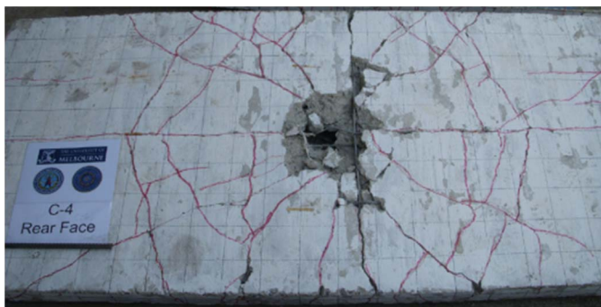
Fig. 6. Crack pattern and concrete spall on rear face of Specimen C4 (Image by G. Tanapornraweekit)
