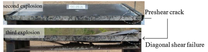
Fig. 20. Shear failure of Specimen GC-2S-2L after third explosion resulting from shear crack initiated during the second explosion (Images by G. Tanapornraweekit)
