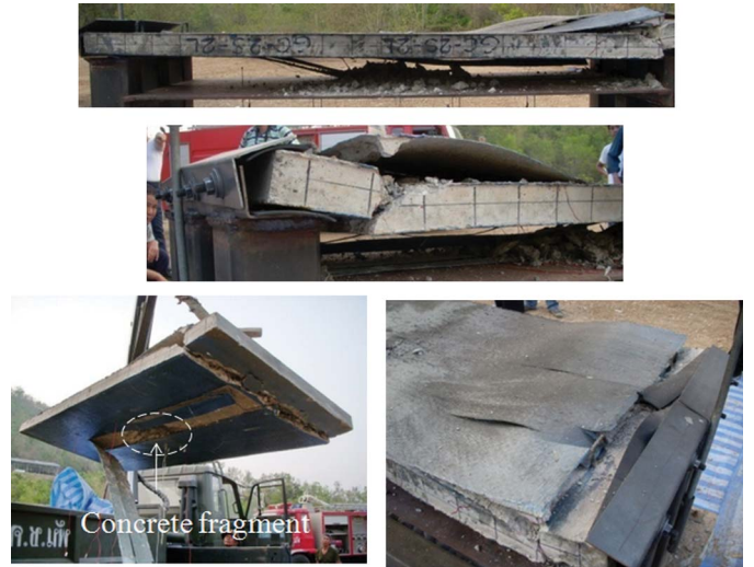
Fig. 19. Failure of Specimen GC-2S-2L after third explosion (Images by G. Tanapornraweekit)
