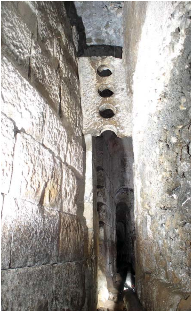
Fig. 6: the stone filter at the entrance of the underground channel of Nemi lake (photo C. Germani).
