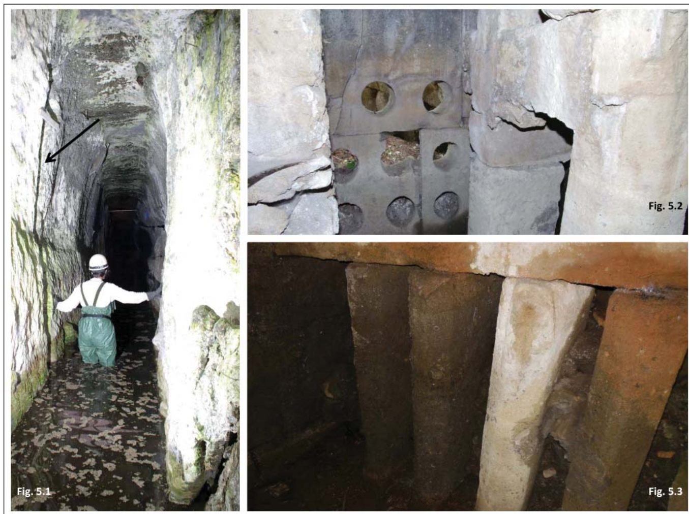
Fig. 5.1: Albano lake emissary: the arrow points to the furrows in the bulkheads. Figs. 5.2 e 5.3: the double stone filter at the entrance of the underground channel of Albano lake (photo C. Germani and P. Bersani).
