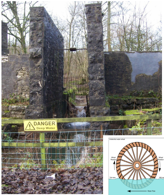
Fig. 10: Water wheel housing at Sedgwick Gunpowder Works; inset illustrates an example of an undershot waterwheel which could have been utilized at Sedgwick.
