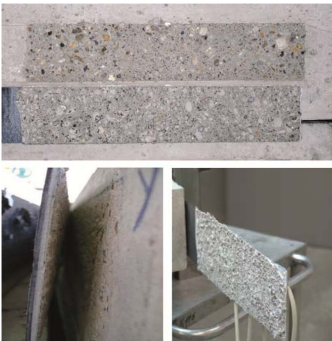
Figure 7. Typical failures due to debonding in the concrete adjacent to the adhesive-concrete interface.
