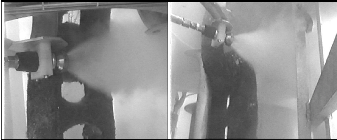
Fig.13. and 14: Cleaning of the chain members by HP water jet
