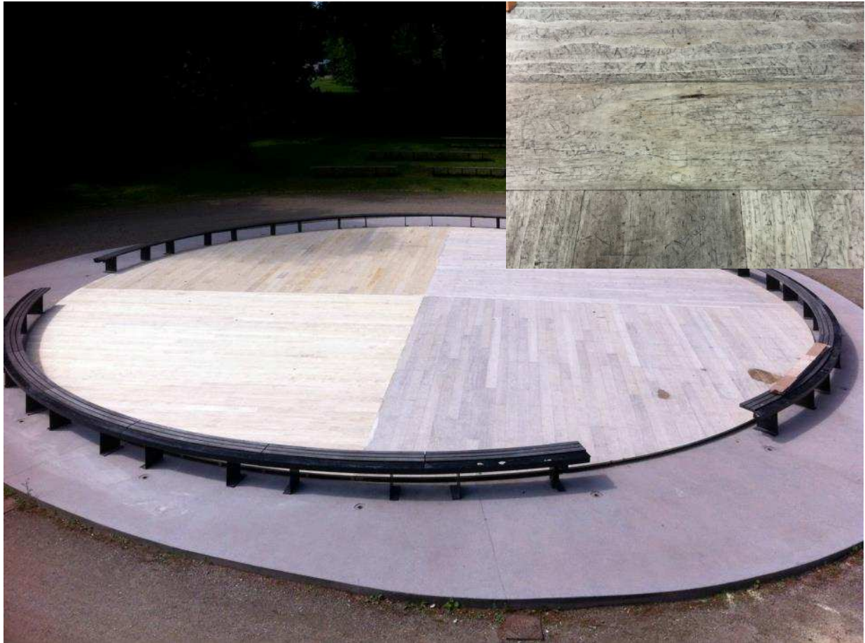
Figure 2: Overview of the exterior dance floor. Picture 3: Close up photo of the surface after 3 seasons before cleaning.
