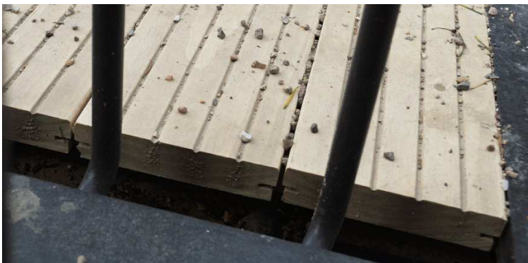
Figure 5: Accoya 34 x 198 mm bridge deck with hidden fasteners.
