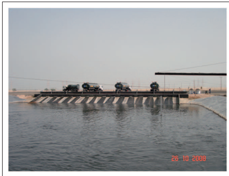
Figure 8. The planned pit is open to receive wastewaters using tanker trucks.
