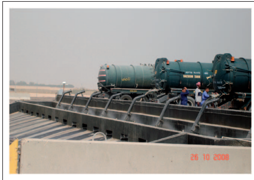
Figure 7. Unloading docking station for the sewage pit as prescribed by the simulation study.
